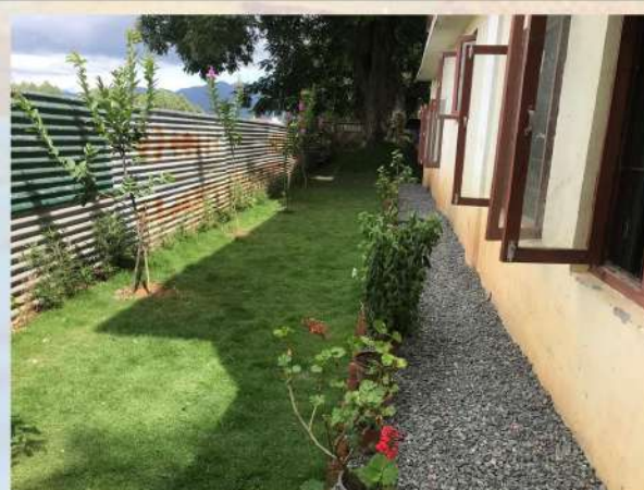
Ground Water Recharge Trench, Shree Balkumari Secondary School
